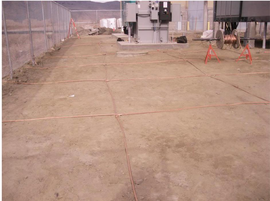
**Copper ground grid before being covered**
