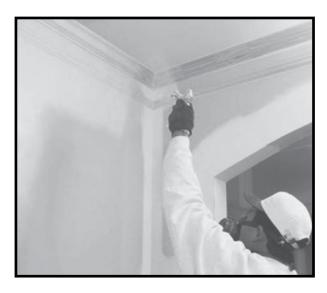
Turn down the pressure as low as it can go while still spraying a good spray pattern to reduce your tip and pump wear. Turning down the pressure also saves paint by reducing overspray.
