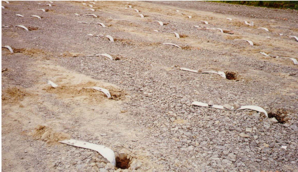
Fig. 4.6 View over site after completed wick drain installation
