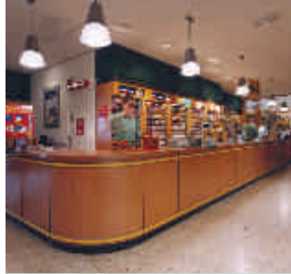
Examples of a recessed-mounted (top) and pendant luminaire
