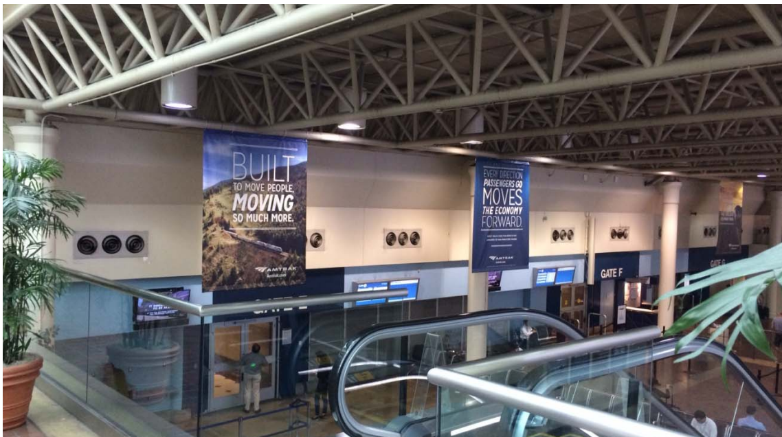
Figure 1. Existing Mechanical Bulkhead
