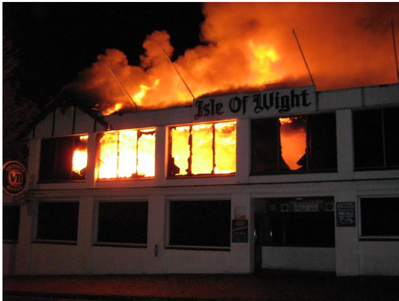
The Isle of Wight Hotel, Cowes was completely destroyed by fire in May 2010.
