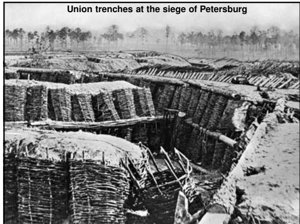
Union trenches at the siege of Petersburg
