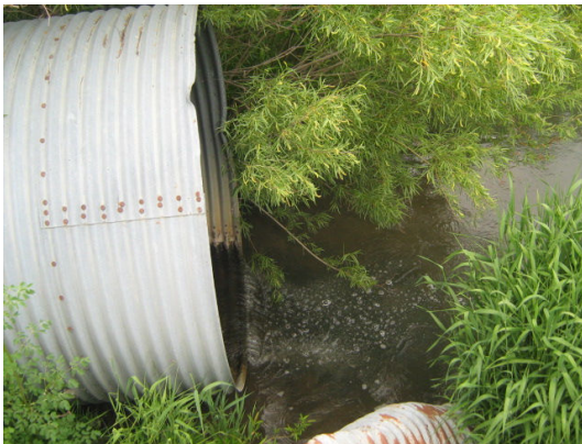
Figure 5-13. Downstream of the Crossing at Beaverton Road.
