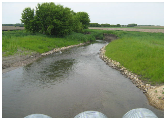
Figure 5-10. Beaver Creek Stream Crossing at HWY 173
