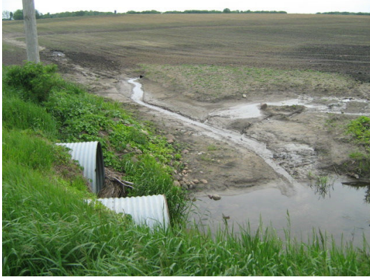
Figure 5-7. Stream Crossing near Intersection of Leroy Center Road and Randall Road.
