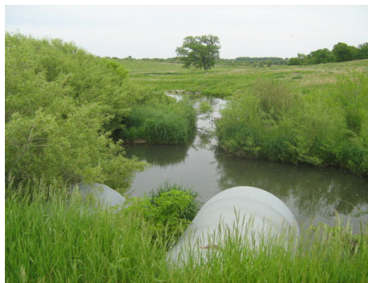
Figure 5-14. Downstream of the Crossing at Beaverton Road.
