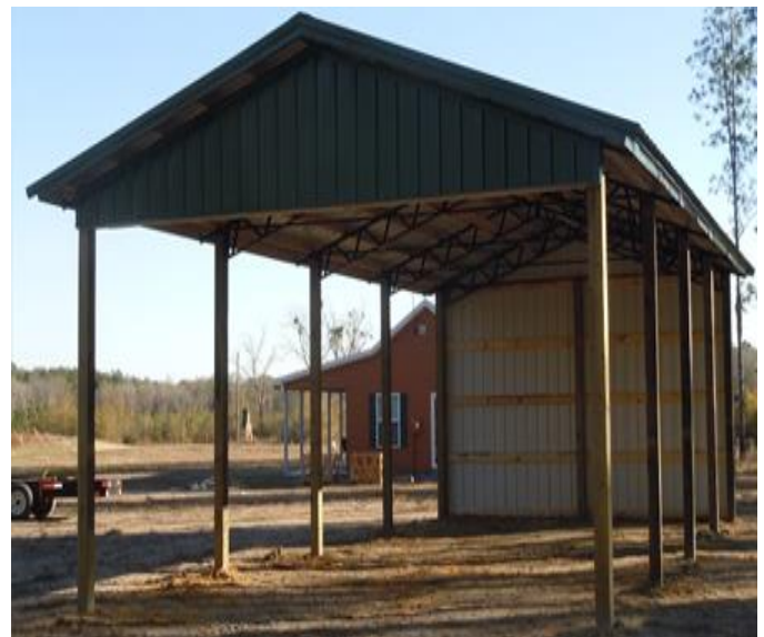
Fig. 2 – Example of open-air storage facility that protects from rain but allows sunlight and air flow among stacked hive bodies containing combs. Photo from Armour Metals, http://www.armourmetals.com/estimate.html .
