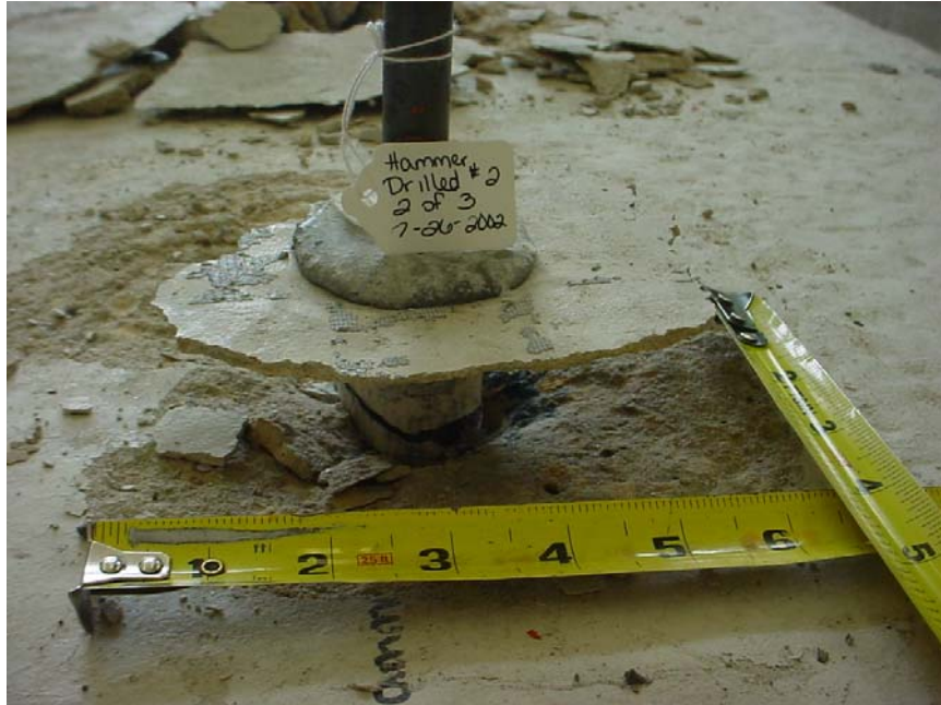
Figure E-5 Typical grout/concrete bond failure of single hammer-drilled anchor with secondary shallow concrete cone and grout plug
