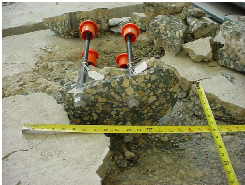
Figure E-10 Typical dissection view of cone failure of quadruple fastener anchor group with anchor spacing of 5 inches
