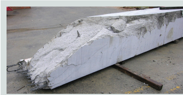
Figure 10. View of LG2 with separated failure surface (outer web face).
