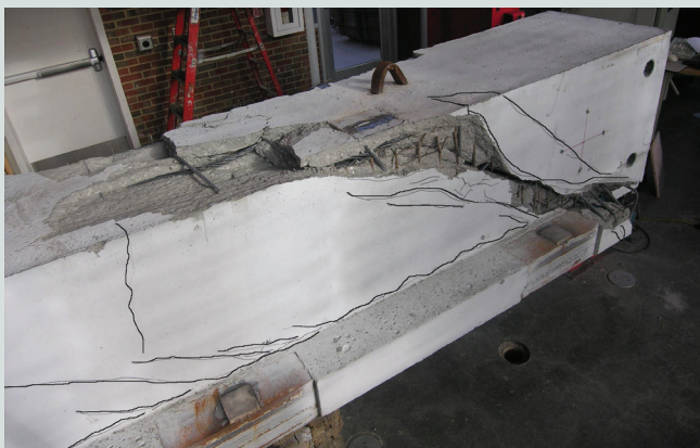
LG3 (U-shaped reinforcing bars across the top)
