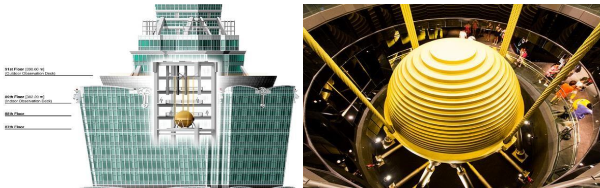
Figure 1. Tuned Mass Damper in Taipei 101.
