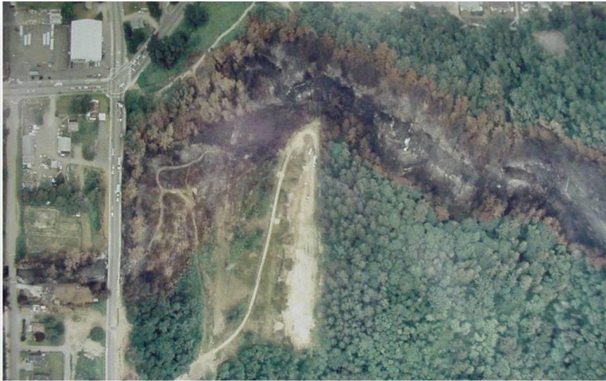
Figure XV - Aerial photo of damage area from 1999 Bellingham Olympic Pipeline rupture and fire.
