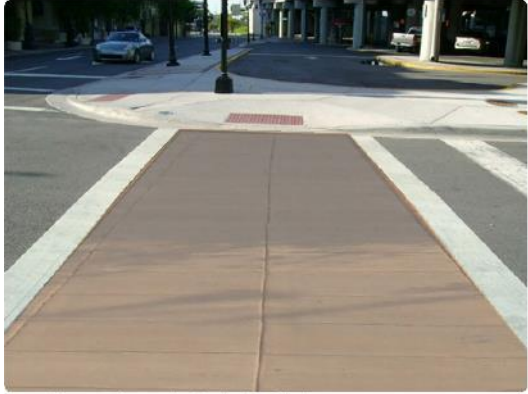
Scored Concrete Crosswalks Bordered with High Visibility Striping. *CityMix 'Omaha Tan' Color Concrete
