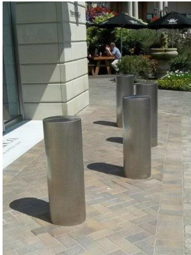
PROPOSED CRASH RATED BOLLARD Calpipe-M-50 Rated Bollard-Storm Cloud Grey Sleeve
