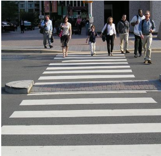
High Visibility Crosswalk: Thermoplastic Striping City Standard Crosswalk Treatment
