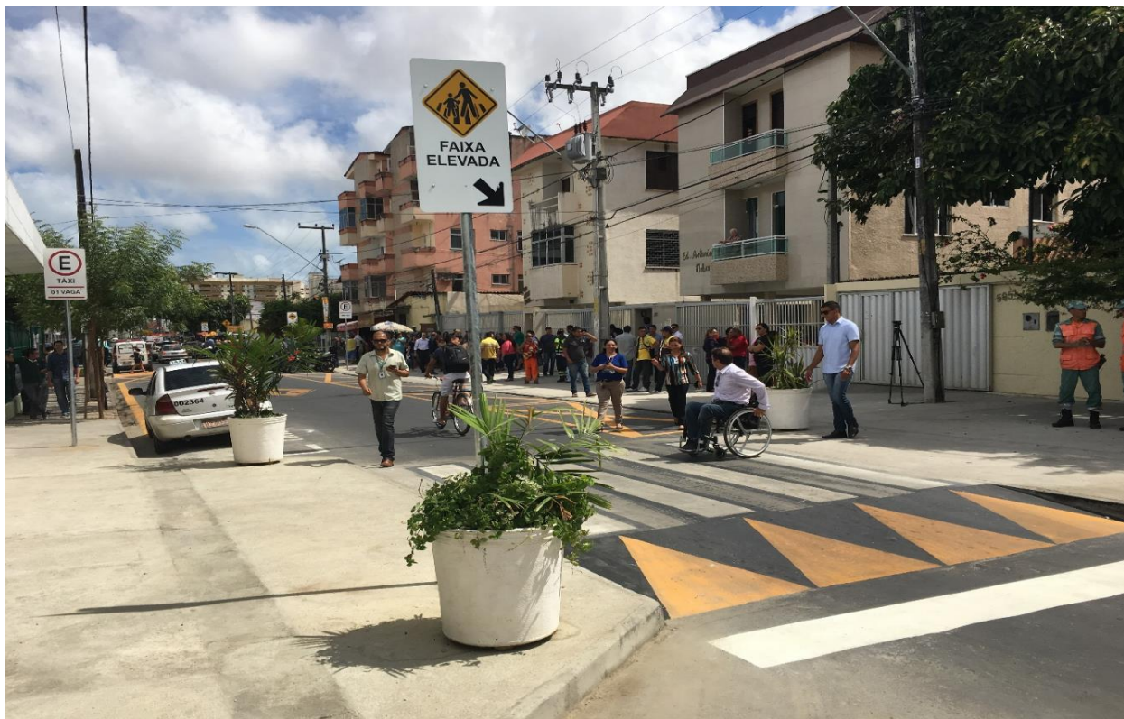
Figure 9. Elevated crossing as part of traffic-calming measures in Fortaleza
