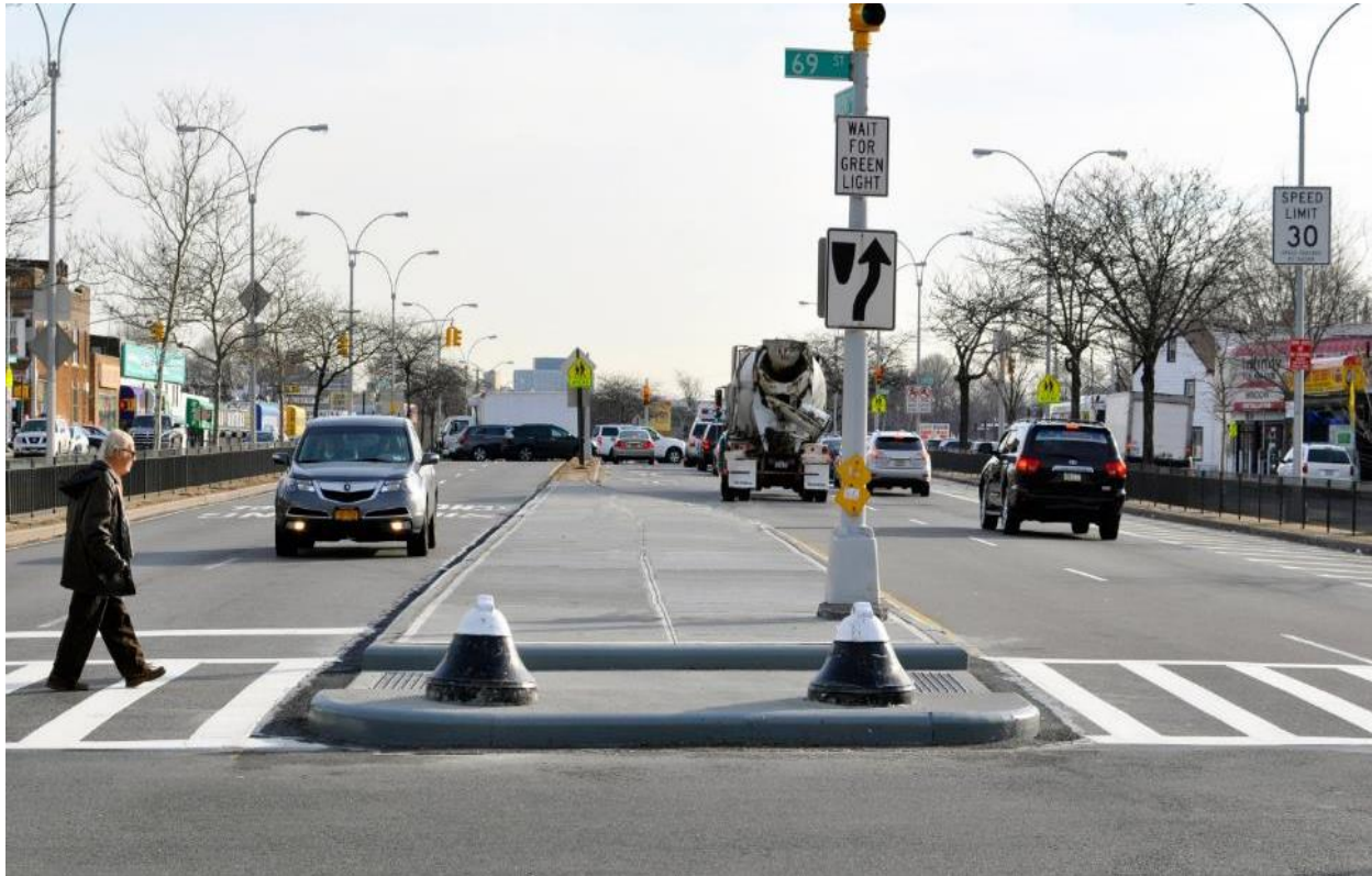
Figure 6. A pedestrian island in Queens in New York City promoting safe crossing
