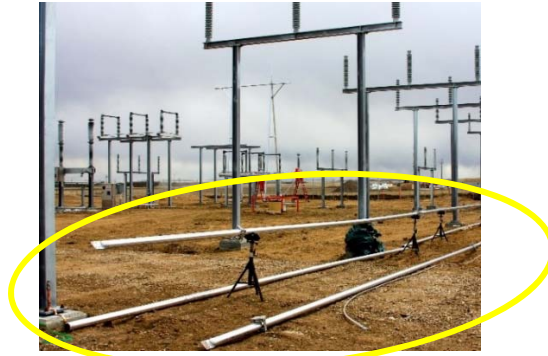
Figure B10 - Equipment Steel Support (TESCO 2013)
