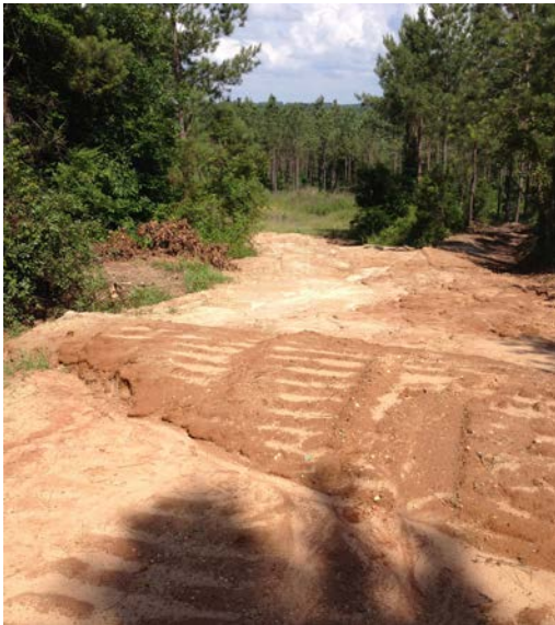
A water bar is a BMP that diverts the flow of water from the road to the forest.
