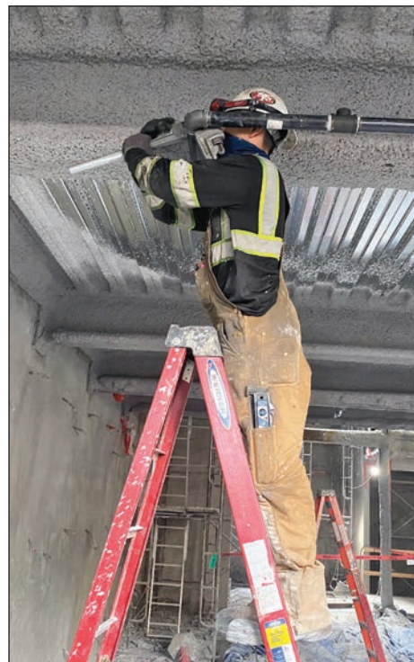
Sprinkler Fitter Apprentice Marcus Gonzales, installs a sprinkler system pipe.
