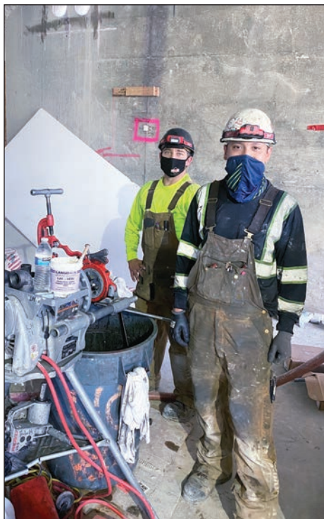
Sprinkler Fitters Vince Copeletti and Marcus Gonzales, on the job.
