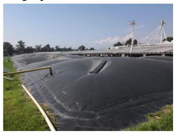
The Topoyanes Farm Wastewater Treatment Plant (WWTP) generates electric power and treated water from swine (hog) dung raised on site. The covered lagoons are built with geomembrane, liner and HDPE (High Density PolyEthylene) cover, and treat the manure from 1 000 pigs.
