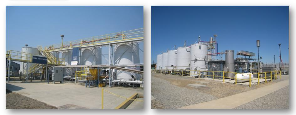
Digester capacity – 3-5 tons per day, Digestion temperature – 125-135 F , Digester volume – 50,000 gal Expected biogas yield –350-583 m<sup>3</sup>/day, Electricity output – 600- 1200 kWh/day Clean World Partners Built the First Commercial Digesters for Food and Paper Waste at American River Packaging, Sacramento
