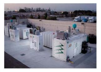
Digester processes 30,000 gal of onion juice per day, Producing biogas containing 70% methane
