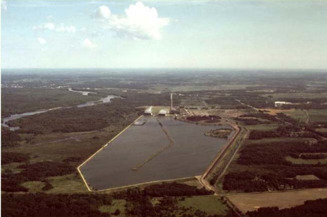
Figure 15: The Wisconsin Power and Light Columbia Plant uses vast quantities of water per hour, and circulates that water in a large cooling lake located immediately next to the plant. Locations like this may present an opportunity for low cost retrofitting for algal carbon capture (Image: Louis J. Maher Jr., University of Wisconsin).
