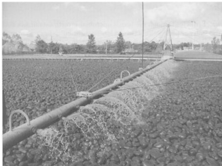
Trickling filters: over rocks (left) and over synthetic media (right)
