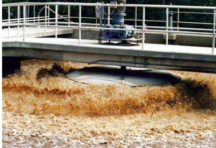
An activated sludge reactor with surface mechanical aeration / oxygen supply at the Stickney Water Reclamation Plant in Chicago
