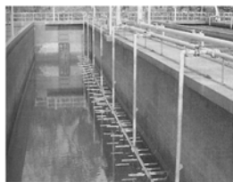
Diffusers near bottom of empty aerator
