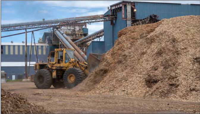
Figure ES-10. This biomass power plant, which has been modified for biochar production and uses forest residues from high fire hazard areas as feedstock, is an example of a centralized biochar production facility. (Photo: Josiah Hunt)
