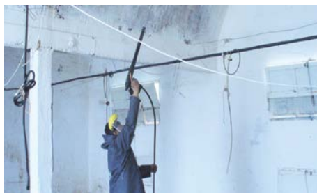
Pressure washing ceiling
