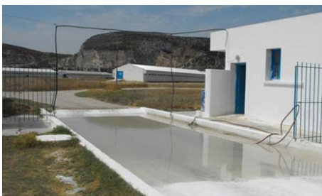
Vehicle disinfection pit
