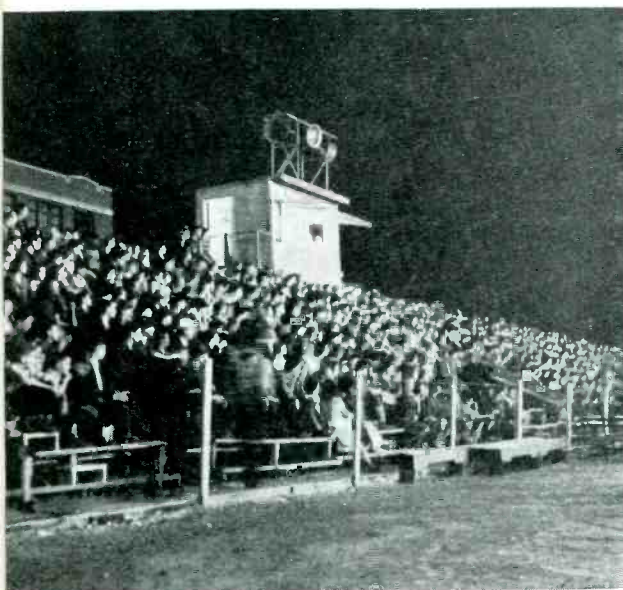
5-YEAR CONTRACT —The Carroll Radio Service, Coffeyville, Kansas, has had the contract to furnish sound to the City's athletic field for the last 5 years. Employs a Clarion 70-100 watt system, finds no difficulty at all in covering up to 5000 people at the games. Does it with 4 speakers mounted on top of press box
