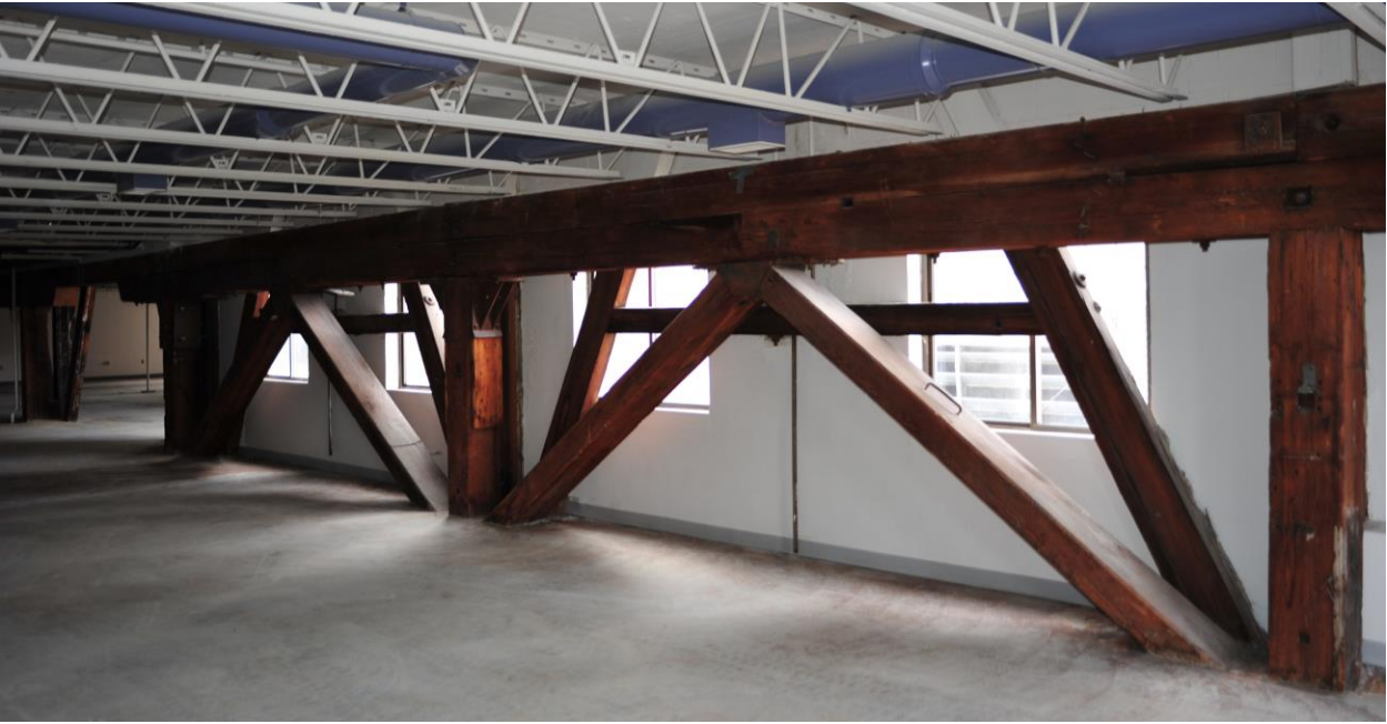
101 Rogers Street, third floor. Craneway framing.
