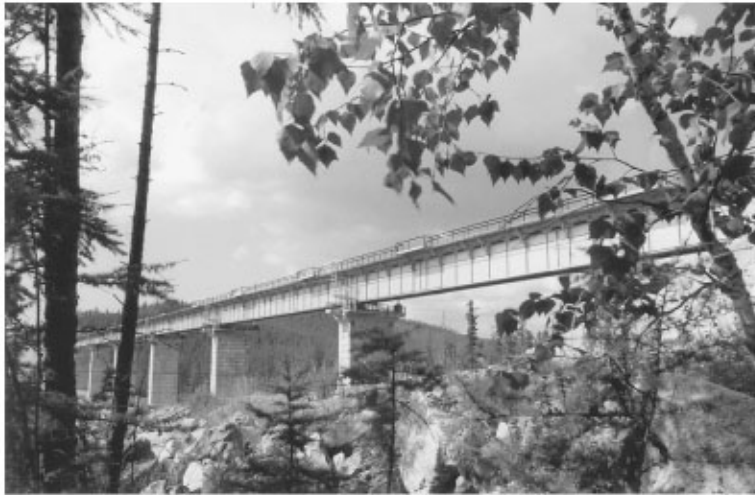
FIGURE 66.8 Deck girder composite bridge of 55 m span over the Mulmuta River (Siberia).
