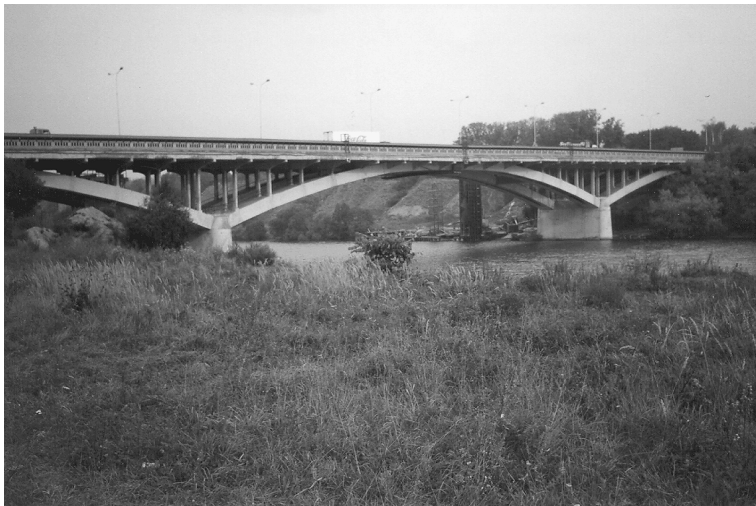
FIGURE 66.35 Moscow Moskva River arch bridge.
