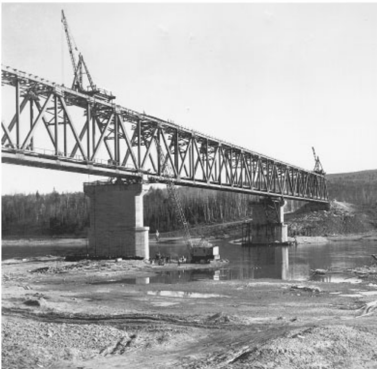
FIGURE 66.12 Cantilever erection of typical truss bridge using derrick cranes.
