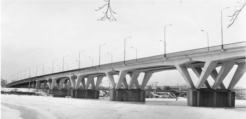
FIGURE 66.32 Penza Sura River Bridge.
