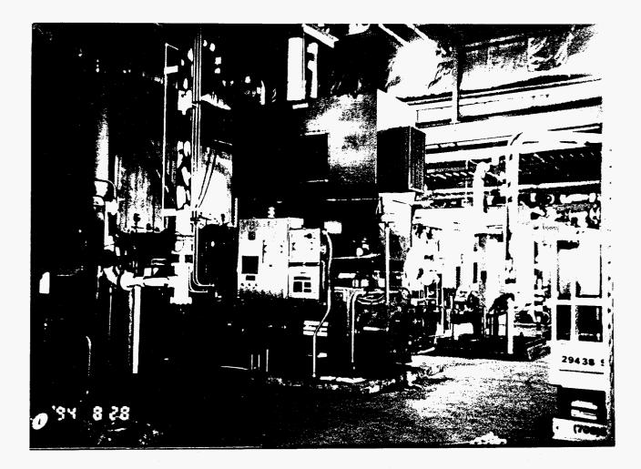
Motor driven, 3 stage, centrifugal air compressor in center. Afterfilters and dryer can be seen in the right background. Construction progress photo, August 1994.
