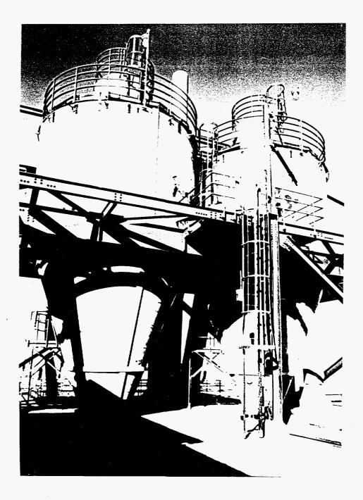
Mill system cyclone separators located on top of the Process Building. Most of the coal is removed from the drying air in these units. Coal flows from the bottom of the separator to the product coal screen inside the building. February 1995.
