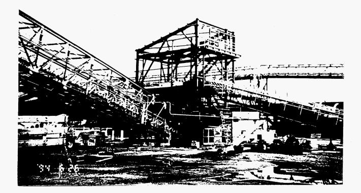
Precrusher building showing reclaim conveyor entering from the right side and plant feed conveyor exiting from the left bottom. Raw coal stockpile conveyor can be seen in the background. Construction progress photo, May 1994.
