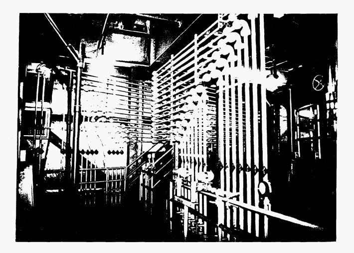
"C" furnace coal injection piping inside the process building. 28 injection pipes are required to supply coal to the furnace. February 1995.
