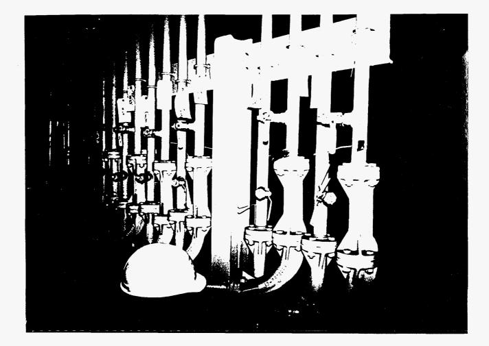
Coal injection piping inside the process building. Special hardened pipe elbows are necessary at each change in coal flow direction. February 1995.
