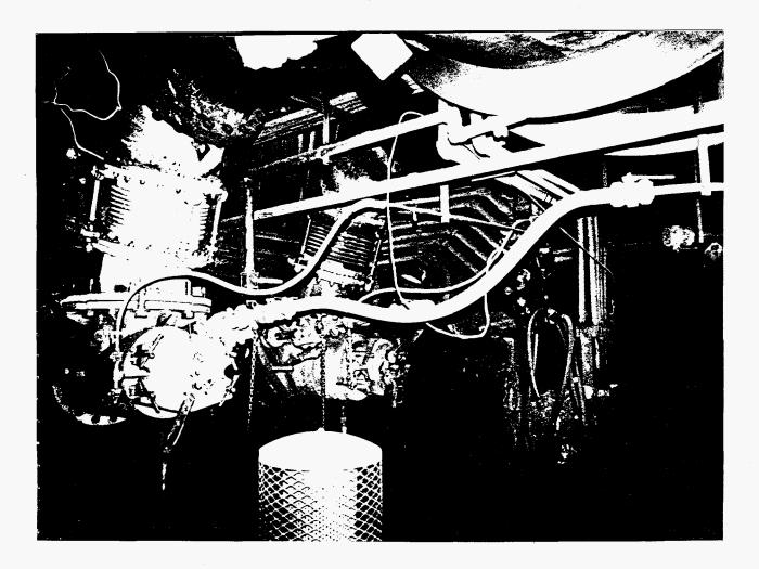
Coal injection flexible hose between the hard pipe on the right and coal injection lance at the blast furnace. February 1995.
