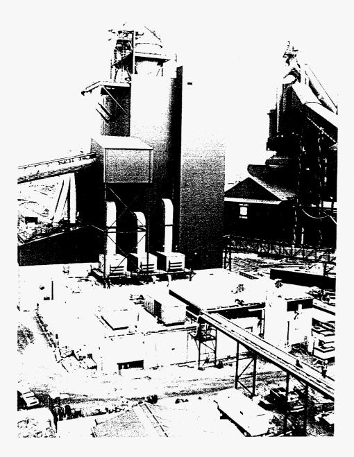
South side of Process Building and Utility Building. Utility pipe bridge enters the Utility Building on the lower right. Note mill system cyclone separators on top of Process Building. "D" blast furnace can be seen to the right of the Process Building. February 1995.
