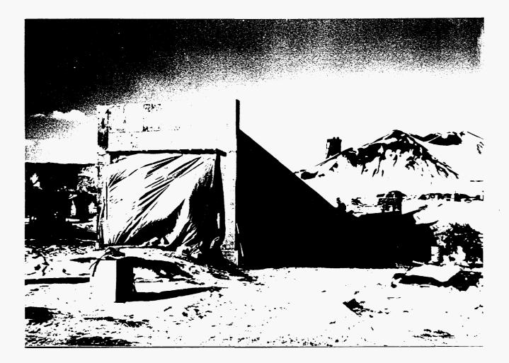
Construction of concrete underground raw coal reclaim tunnel prior to placing soil back fill material which will cover all but the tunnel opening in the foreground. Tunnel is 12' wide x 16' high x 400' long. Construction progress photo, January 1994.
