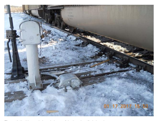
Figure 4. Accident switch and pieces of the long-handled shovel.
