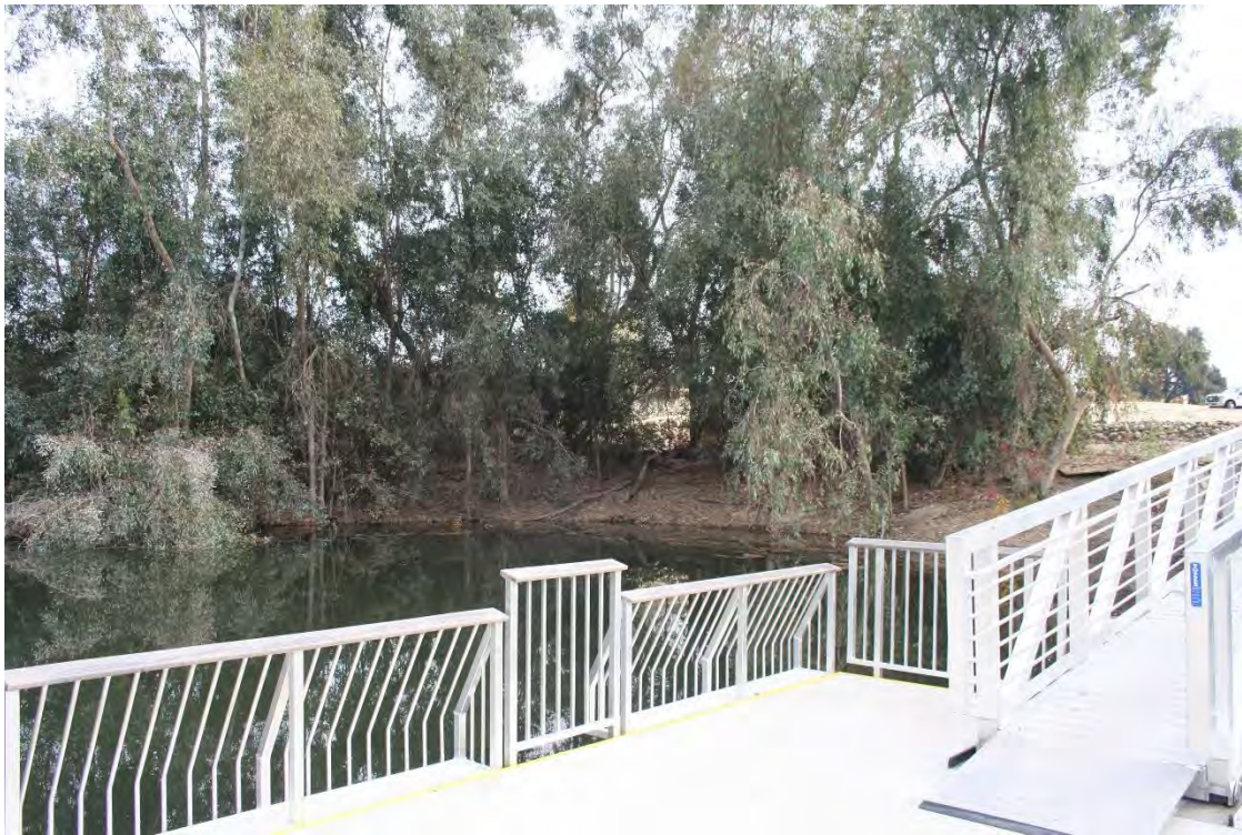
Figure 4: Fishing Pier after water level increase from installation of the French Drain.
