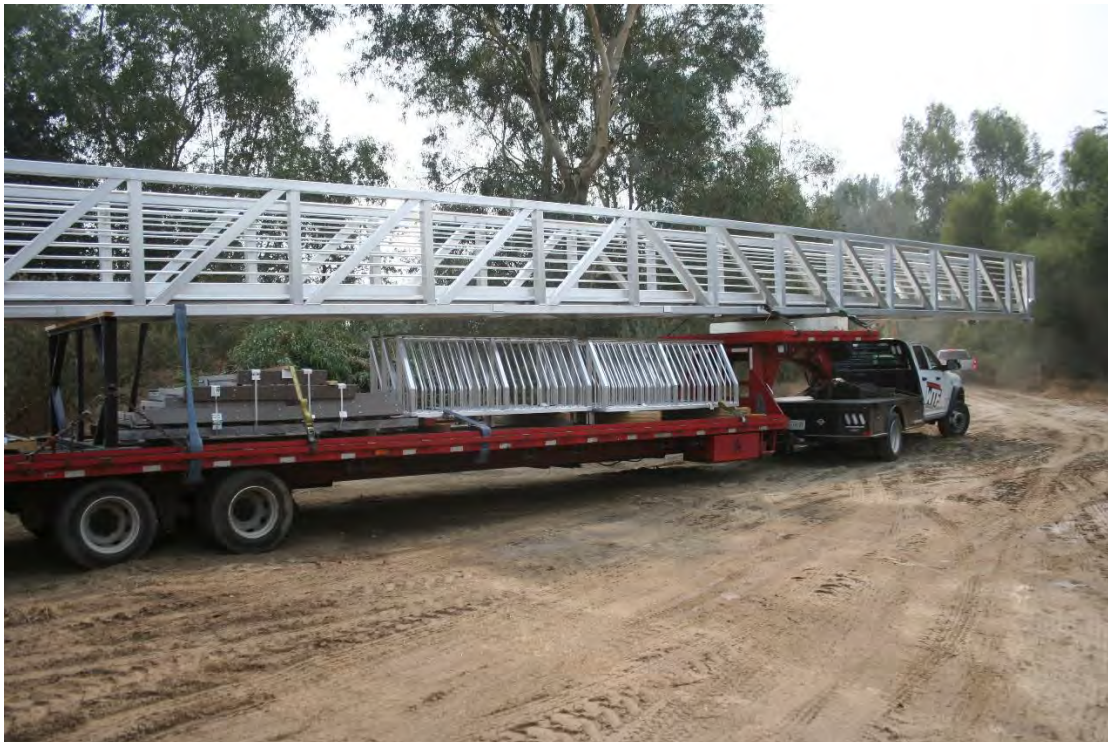
Figure 5: Delivery of the 88-foot gangway.
