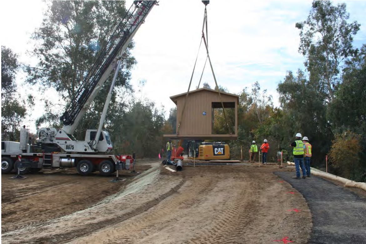
Figure 8: Installation of the vault restrooms.
