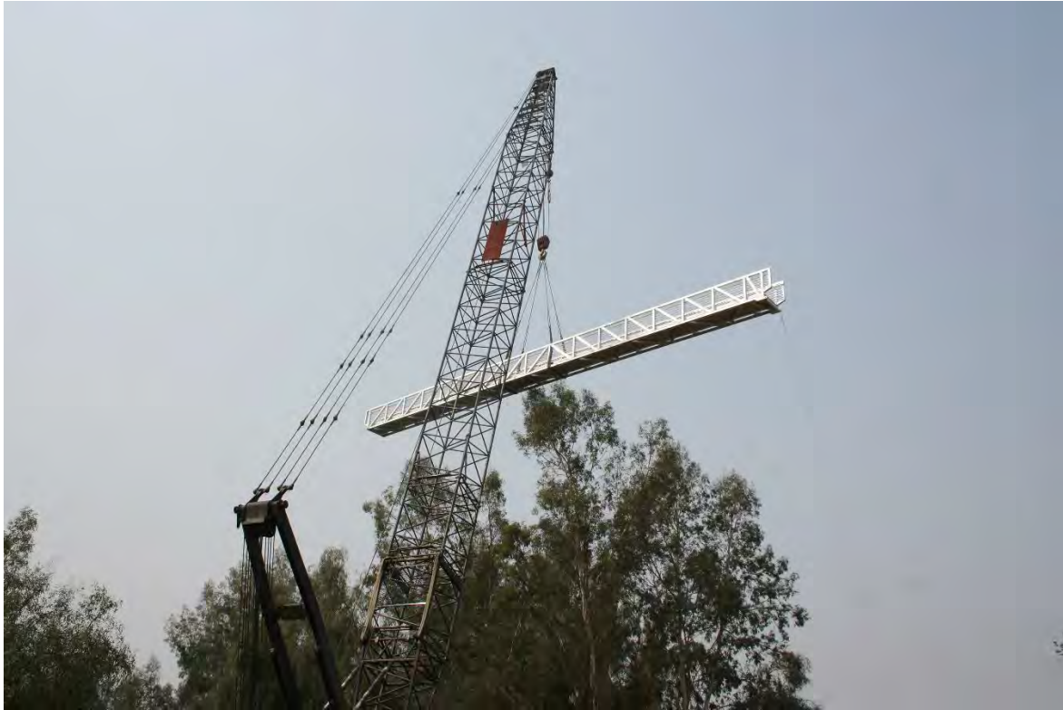
Figure 6: Installation of the gangway
