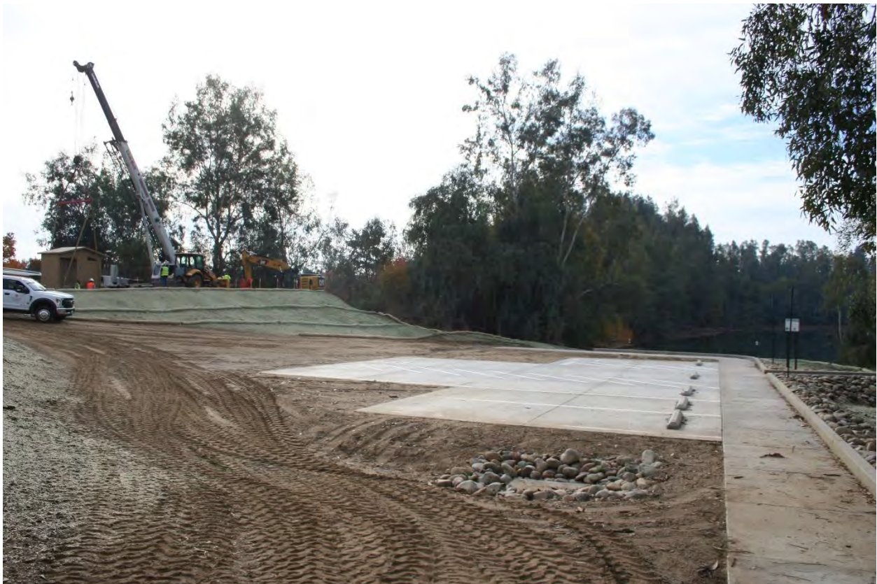
Figure 7: Concrete and gravel parking area.
