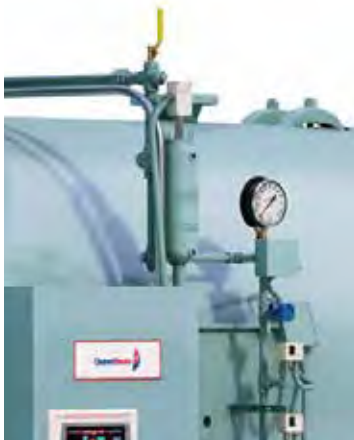
Figure 1-27: Water Column and Vent Valve
