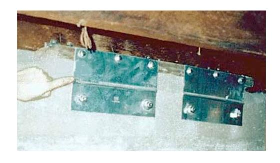
anchors" are used to secure the house to the foundation.
