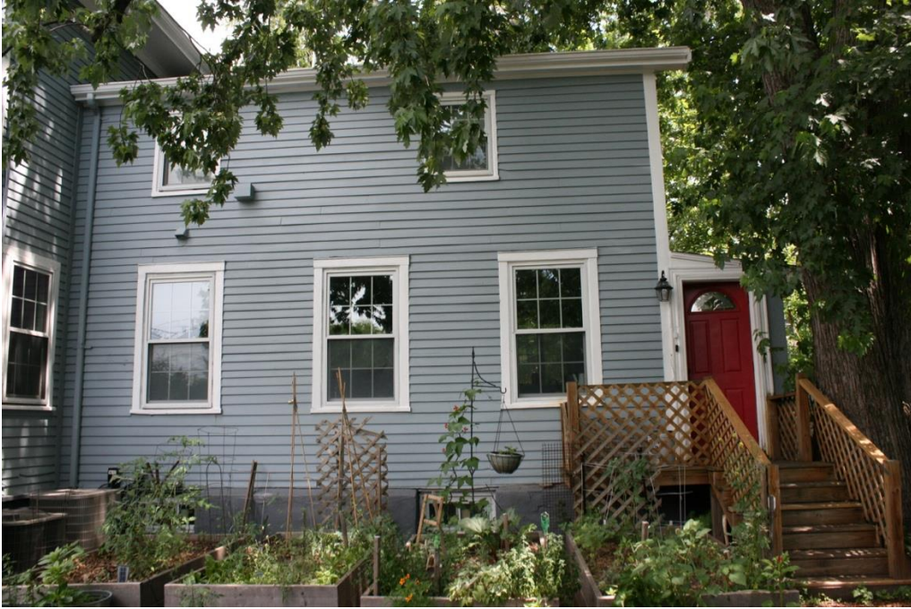
Figure 6. Ell, rear (southwest) elevation.
