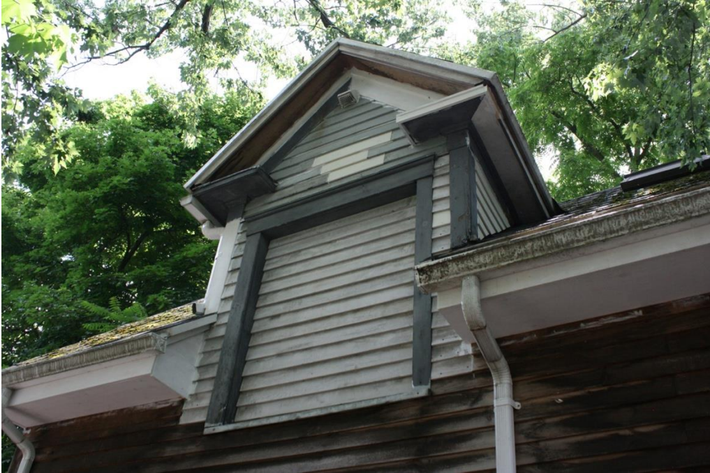
Figure 14. Carriage house facade, dormer window detail.
