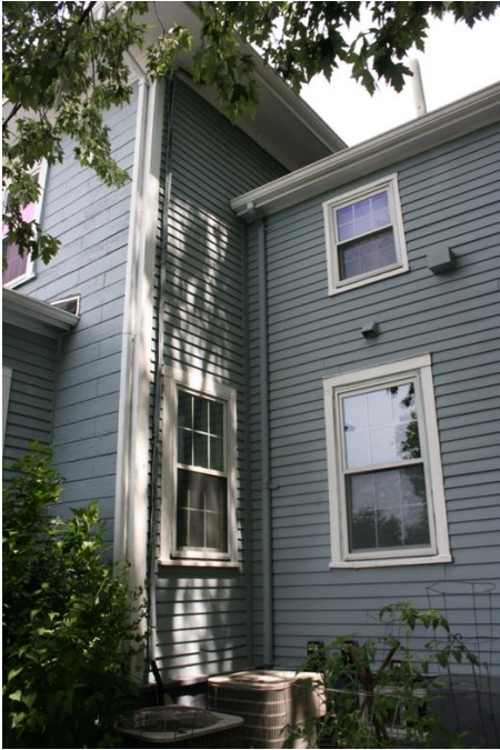
Figure 5. Main house, southeast side elevation.
