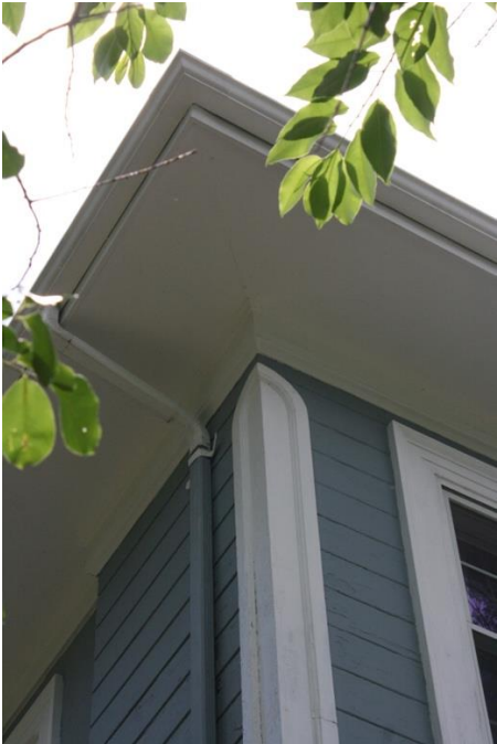
Figure 11. Main house, eave detail.
