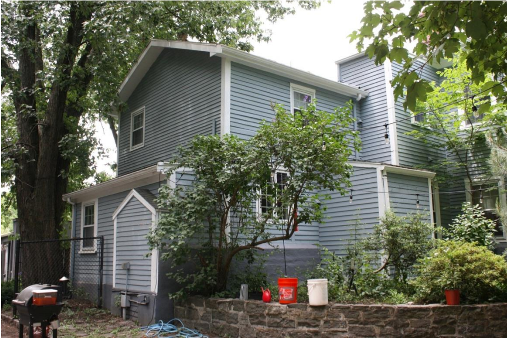
Figure 7. Ell, side (southeast) and front (Logan Street) elevations.
