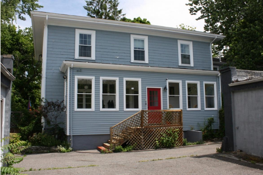
Figure 4. Main house, rear (southwest) elevation.
