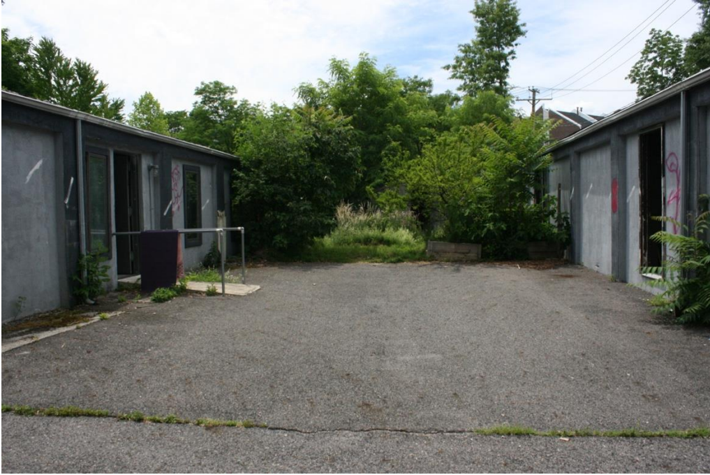
Figure 16. Middle (L) and west (R) garage buildings (demolished 2021).
