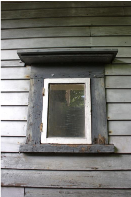
Figure 15. Carriage house, window detail on southwest elevation.
