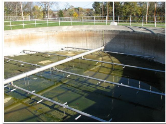
Existing WAS Holding Tanks
