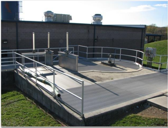
The Existing Grit Chamber
