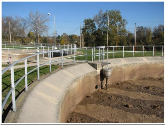
Existing WAS Holding Tanks
