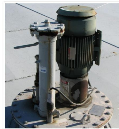
Floating Cover on the Existing Primary Digester (1 of the 2) Existing Mixing Pumps
