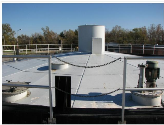
Floating Cover on the Existing Primary Digester (1 of the 2) Existing Mixing Pumps
