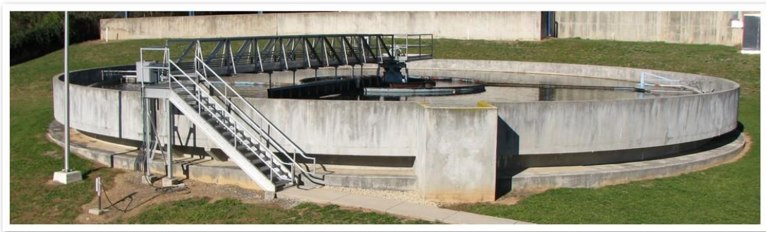
(1 of 3) Existing Final Clarifiers
