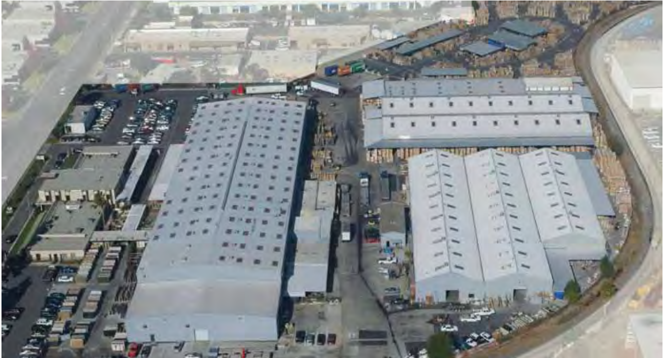
Aerial View of MSI Corporate Headquarters Orange, CA
