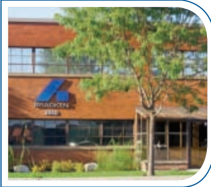
Pattern, casting and machining facilities located in London, Ontario Canada (Single Source Solutions)
