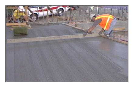
Figure 2.2-2. Finisher Checking the Freshly Placed Deck Concrete Near the Expansion Joint Blockout.
