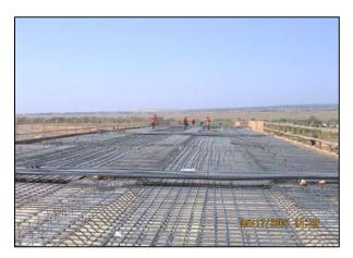
Figure 3.2-2. Truss Bars Must Not be Allowed to Rotate out of Vertical.
