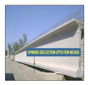
Figure 4.1-3. Measuring for Precast, Prestressed "I" Girder Camber.
