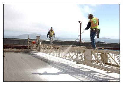
Figure 6.2-1. Applying Spray Cure from a Moveable Bridge Following the Finishing Machine.
