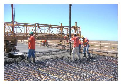
Figure 5.3-1. Vibrating Concrete.
