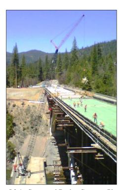
Figure 5.2-1. Crane and Bucket Concrete Placement.
