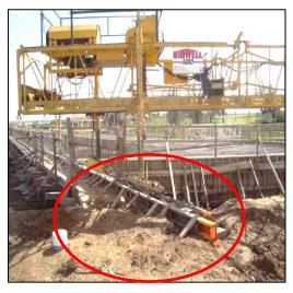
Figure 4.2-2. Screed Rail Should Extend Beyond Pour Area.
