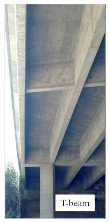
Figure 2.1-6. Example of a T-Beam Bridge.
