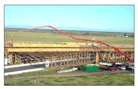
Figure 5.2-2 Concrete Pump.
