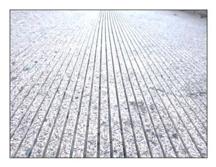
Figure 6.1-7. Close-up of Grooving.
