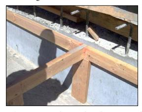
Figure 2.1-1. Typical Deck Form Support for a Concrete Box Girder Bridge.
