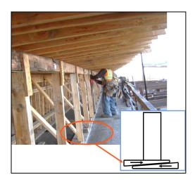
Figure 4.2-1. Wedge System for the Overhang.
