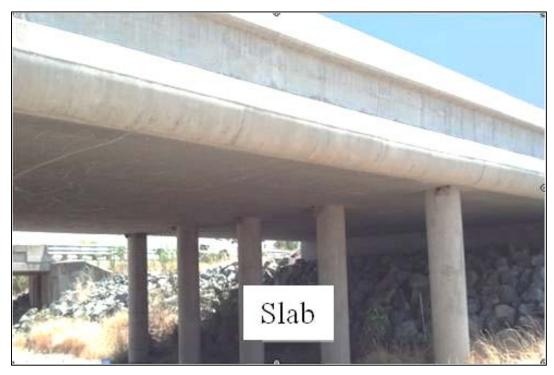
Figure 2.1-4. Example of a Slab Bridge.
