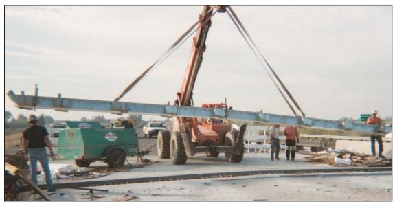
Figure 2.2-4. Joint Seal Assembly Installation.
