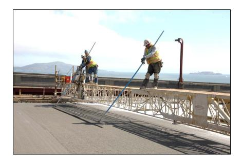
Figure 6.1-6. Longitudinal Tining Typical Process.
