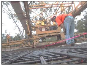
Figure 4.2-5. Check Finishing Machine Height.
