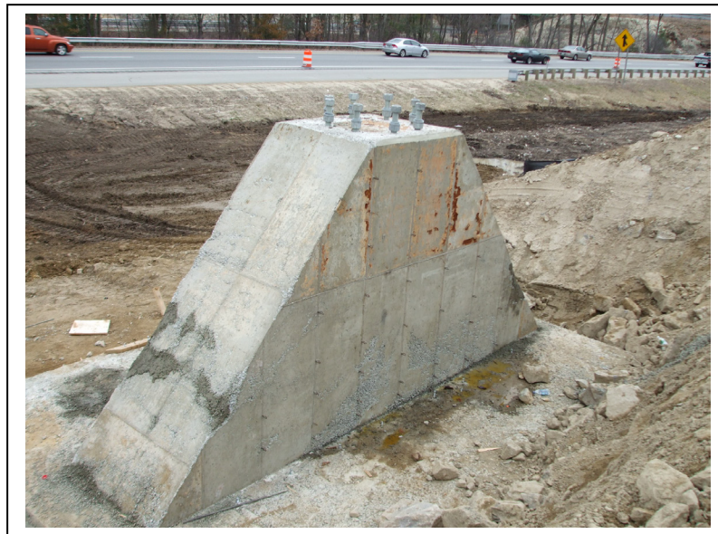
Typical NHDOT Sign Structure Footing
