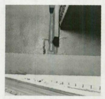
(b) Cracking at transverse diaphragm web connection plate (skewed bridge)
