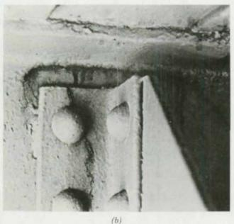
Fig. 43. Crack in stringer web above a web bracket
