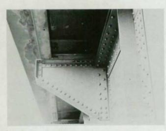
Fig. 68. Cantilever bracket showing web connection
