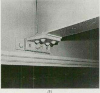
Fig. 54. Diaphragm with missing bolts in end connection
