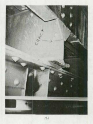
Fig. 44. Web cracking at cut-short web stiffener
