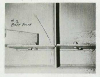
Fig. 58. Cracked web at end of lateral gusset plate (note separate plates are not connected to stiffener)
