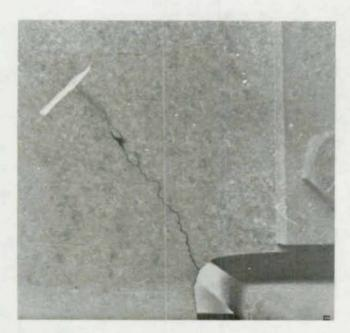
Fig. 38. Cracked web at simple stringer end connection from restraint and reduced bending resistance
