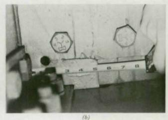
Fig. 55. Cross-frame detail which has developed fatigue crack growth
