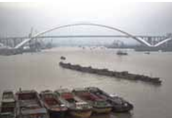
Figure 8 The Lupu Bridge in China, built from steel and concrete and opened in 2003 was the longest through arch bridge in the world until 2009. ( http://en.wikipedia.org/wiki/File:LupuBridgeandBoats.jpg )
