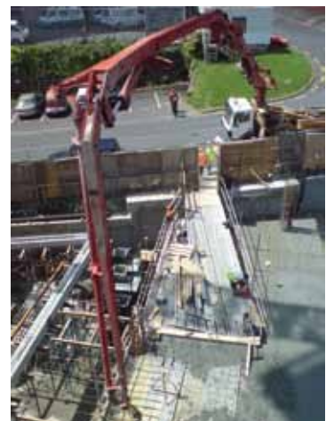
Figure 5 – A pump may be used to move concrete to an elevated position or a difficult to reach area. ( http://upload.wikimedia.org/wikipedia/commons/a/a0/Concrete_Pump_At_Works_Site.jpg )
