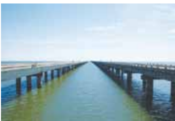
Figure 4 Lake Pontchartrain Causeway Bridge in Louisiana, USA ( http://www.creativesuite.com/cities-landscapes/5-longest-bridges-in-the-world )
