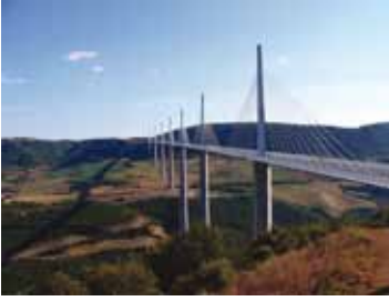
Figure 5 The Millau Viaduct across the Tarn Valley in France is a multiple span cable-stayed consisting of eight spans supported by seven towers. ( http://dannyoigrady.com/images/millau-viaduct-france.jpg )
