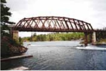
Figure 1 The original Sioux Narrows Bridge in Ontario Canada. A wooden truss bridge built in 1936 from Douglas fir. ( http://www.flickr.com/photos/77136894@N00/2334314530/ )
