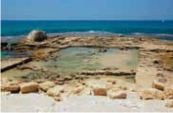
Figure 1 – The Roman baths at Caesarea built from Roman concrete which would set underwater. ( http://en.wikipedia.org/wiki/File:Caesarea_Concrete_Bath.jpg )
