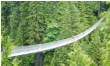
Figure 2 The Capilano Bridge in Canada is an example of a simple suspension bridge in which the deck is supported by the hand rail cables. ( http://en.wikipedia.org/wiki/File:CapilanoBridge.jpg )
