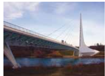
Figure 4 The Sundial Bridge in California is an example of a cantilever-spar cable-stayed bridge. ( http://en.wikipedia.org/wiki/File:Sundial_Bridge_at_Turtle_Bay.jpg )
