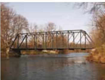
Figure 3 Through truss bridge where road sits under truss. ( http://www.historicbridges.org/truss/mckeowen/ )
