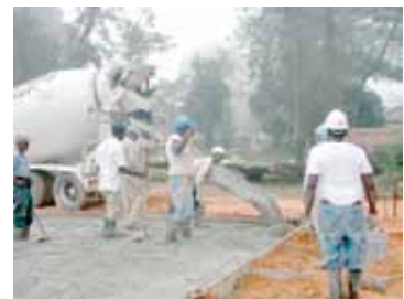
Figure 4 – Pouring a concrete raft for the floor of a building. ( http://upload.wikimedia.org/wikipedia/commons/5/58/Concrete_pouring_0020.jpg )
