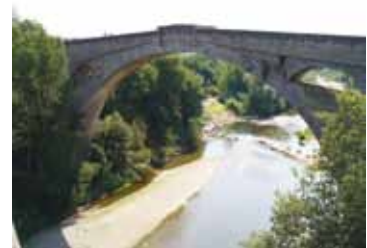
Figure 5 The Pont du Diable in France is an early example of an open spandrel bridge. ( http://en.wikipedia.org/wiki/File:Pont_du_Diable_2.JPG )
