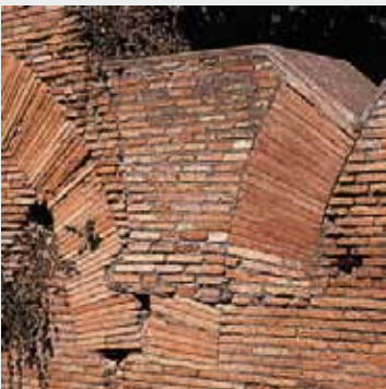
Figure 3 - The Romans used mobile kilns to make bricks where ever they went. This is a fine example of a Roman brick wall with embedded arches. ( http://www.architectureweek.com/2005/0803/images/surfaces_B129 ).
