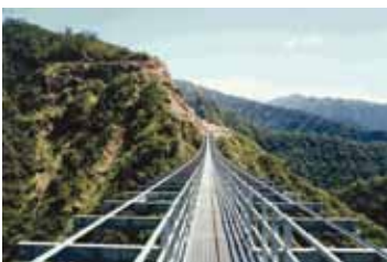
Figure 3 The Arroyo Cangrejillo Bridge in Argentina is the longest simple suspension bridge in the world with a span of 337 metres. ( http://www.ketchum.org/Cangrejillo/fig15-700x470.jpg )
