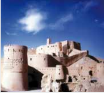
Figure 1 - The Arg-e Bam citadel in Iran was the largest adobe structure in the world until it was destroyed by an earthquake in 2003. This is just one small part of the huge, sprawling complex that was built 2500 years ago. ( http://en.wikipedia.org/wiki/File:Arge_Bam_Arad_edit.jpg )
