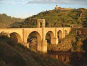
Figure 1 The Roman arch bridge at Alcantara constructed from concrete and clad in brick. ( http://en.wikipedia.org/wiki/File:Bridge_Alcantara.JPG )
