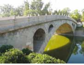
Figure 6 The Zhaozhou Bridge in China is the oldest surviving example of an open spandrel segmental arch bridge. ( http://en.wikipedia.org/wiki/Zhaozhou_bridge )
