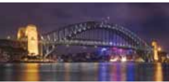
Figure 7 Sydney Harbour Bridge is a well known example of a through arch bridge. The main arch is 503 metres wide and 139 metres tall. The deck is 49 metres wide and has a clearance of 49 metres above the water. ( http://en.wikipedia.org/wiki/File:Sydney_Harbour_Bridge_from_Circular_Quay.jpg )
