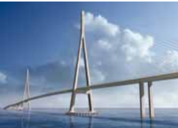
Figure 6 The Sutong Bridge over the Yangtze Rver in China has the longest cable-stayed span in the world at 1.088 kilometres. ( http://www.lqgcs.com/uploads/allimg/200909/1-0Z919141537.jpg )
