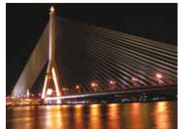
Figure 3 The Rama VIII Bridge in Thailand has only one supporting tower located to one side of the centre of the span. ( http://en.wikipedia.org/wiki/File:Rama_VIII_Bridge_at_night.jpg )
