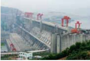
Figure 6 – The Three Gorges Dam in China holds the world record for the largest concrete pour in a single project. ( http://upload.wikimedia.org/wikipedia/commons/7/7c/Dreischluchtdamm_hauptwall_2006.jpg )
