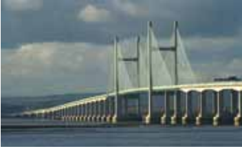
Figure 5 The Second Severn Crossing ( http://www.flickr.com/photos/beimages/175286033/ )
