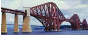
Figure 2 Forth Railway Bridge in Scotland constructed entirely from steel and holding the record for the longest cantilever bridge for 17 years. ( http://www.edinburghvilla.com/EdinburghForthRailBridgecrop2.jpg )
