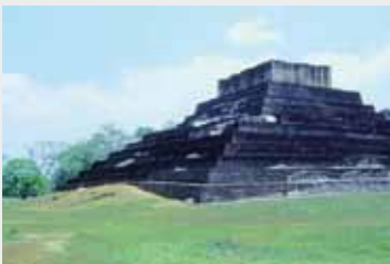
Figure 2 The Mayans used fired bricks made from clay to build the city of Comalcalco as no stone was available locally. ( http://www.mexconnect.com/articles/1241-did-you-know-mayan-pyramid-in-tabasco-mexico-has-possible-roman-links )
