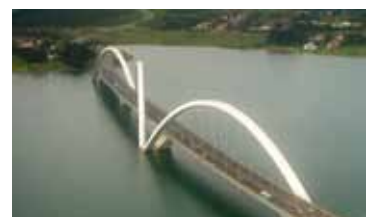
Figure 4 Juscelino Kubitschek Bridge over Lake Paranoá in Brazil ( http://en.wikipedia.org/wiki/Juscelino_Kubitschek_bridge )
