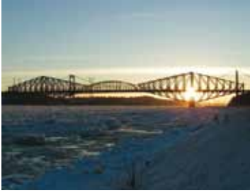
Figure 6 The Quebec Bridge over the Saint Lawrence River in Canada – the longest truss bridge in the world ( http://www.creativesuite.com/cities-landscapes/the-quebec-bridge )
