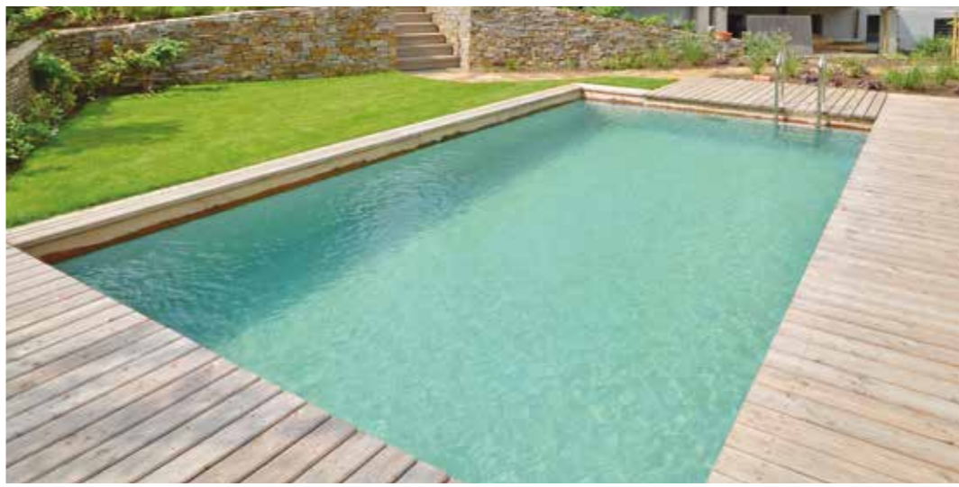
Living-Pool The pure form of the Living-Pool. Looks just like a conventional facility, but features exclusively biological water treatment.
