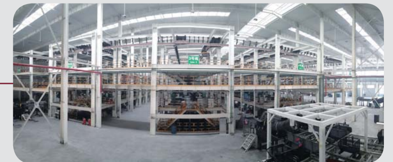
Threading, Air Pressure Test, and Anti-rust Treatment
