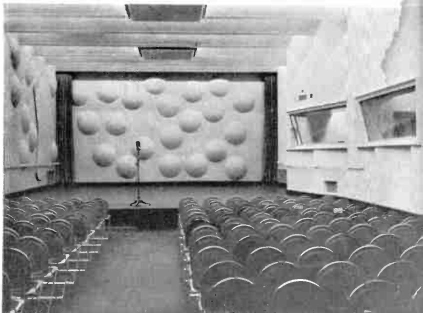
Below: A modern broadcasting studio (NBC, New York, 1945). The spherical protuberances at the back and side of the stage are functional, designed to aid in the diffusion of reflected sound.
