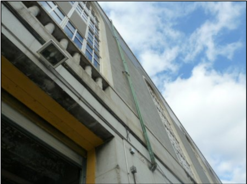
Vent pipe for reported former UST
