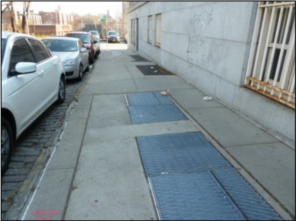
Transformers along sidewalks
