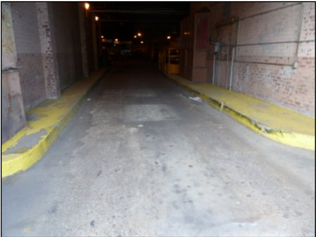
Reported location of former UST
