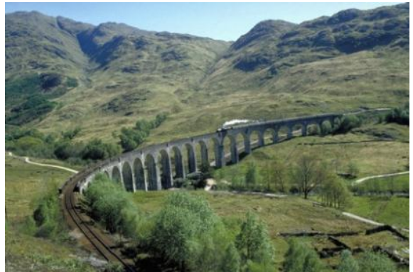
The Glenfinnan Viaduct in Scotland bore the Hogwarts Express (really the Jacobite Steam Train) and its students to magic school!
