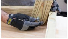
Install the washer and wingnut to secure the angled supports.
