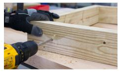
Using a %" drill bit, make a hole at this point.
