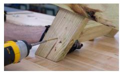
Use two 2  $\frac{1}{2}$ " wood screws at each end to attach part (D) to parts (C).
