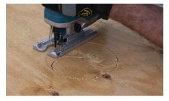
Insert the jigsaw blade into this hole and proceed to cut out the circle.
