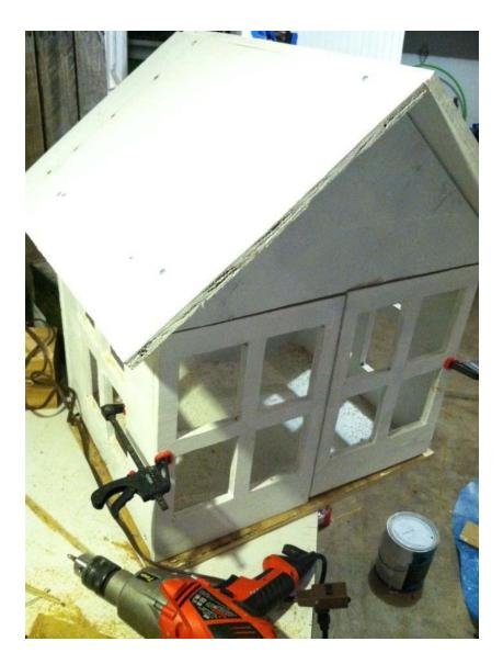
7. **Get Roofing!** Slather the top with wood glue. Use cedar shims to elevate the look to another level! The cedar slats were cut between 6 1/2'' inches to 7 1/2'' in varying lengths to make it look more authentic. We used three rows of the cedar "shingles". The cedar roof provides another layer of protection from the weather. (on our to-do list – seal the cedar roof with a clear sealer)
