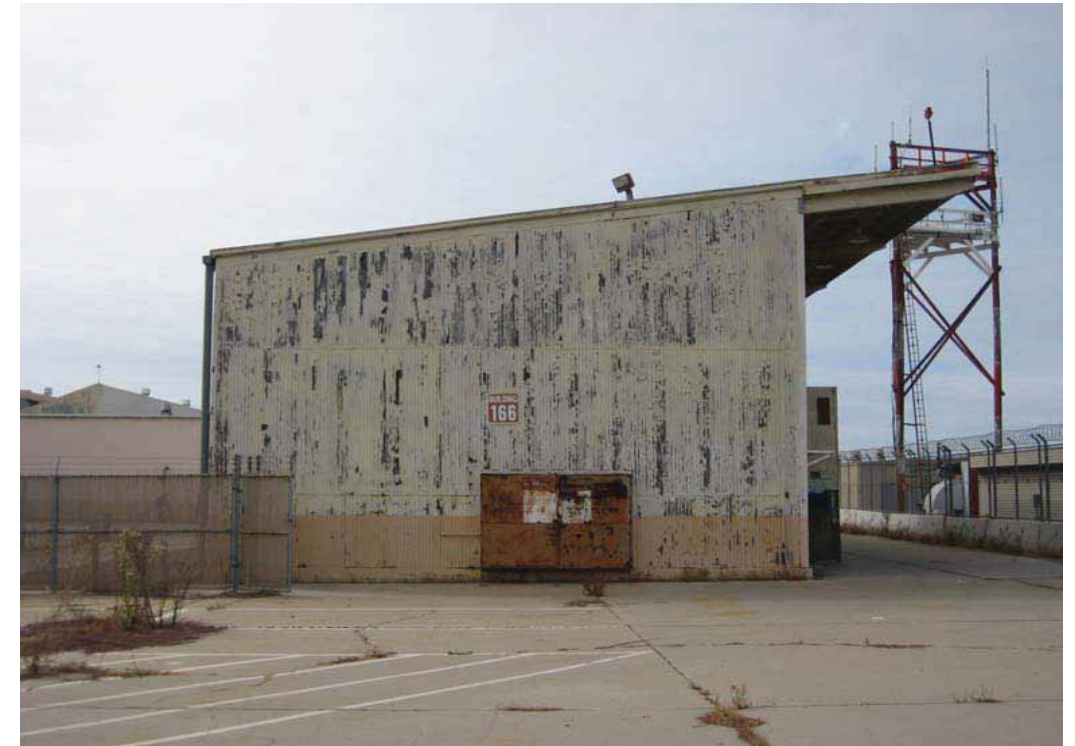
Building 166 - Salvage Headquarters, East Elevation, San Diego, California, October 2009.
