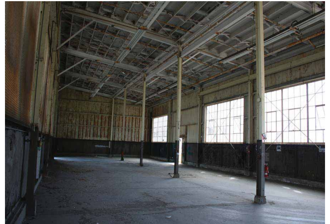
Building 166 - Salvage Headquarters Interior, facing Southeast, San Diego, California, October 2009.
