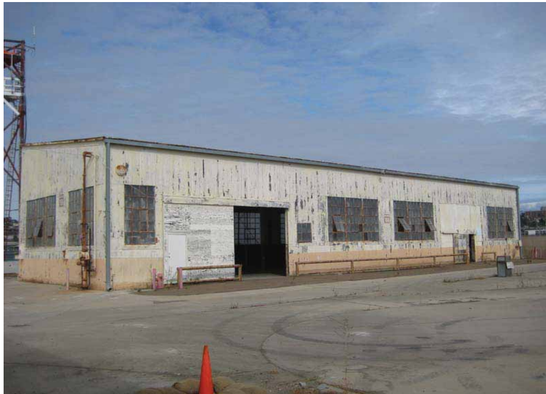
Building 166 - Salvage Headquarters, Southwest Oblique, San Diego, California, October 2009.
