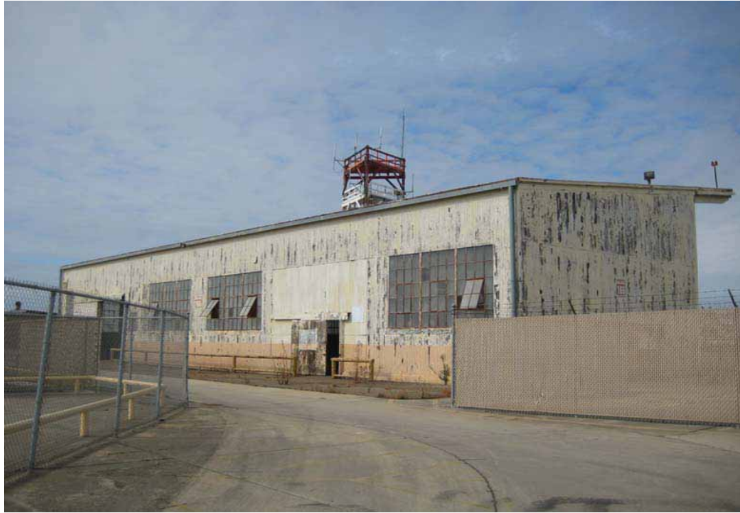
Building 166 - Salvage Headquarters, Southeast Oblique, San Diego, California, October 2009.
