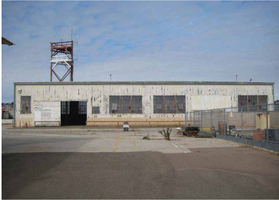
Building 166 - Salvage Headquarters, South Elevation, San Diego, California, October 2009.
