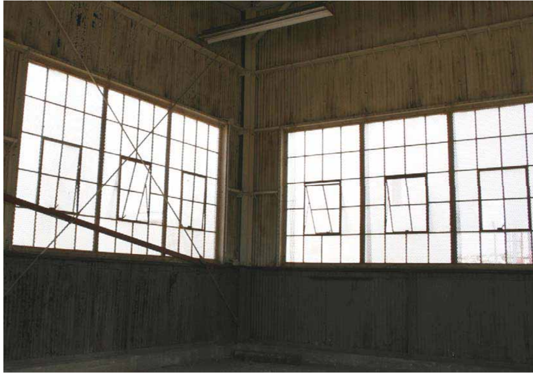
Building 166 - Salvage Headquarters Interior, facing Northwest, San Diego, California, October 2009.
