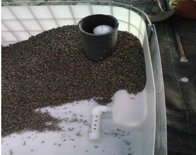
Utelite Expanded Shale for the Gravel - - - - - Bell Siphon installed
