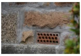
Some patch repairs have been undertaken to the pointing during the history of this dwelling. Where the entrance door is located originally there was some ornate cornicing immediately above the door, similar to that on No. 34, but this has obviously long since cracked and broken away, there now being a light scar on the granite where this was originally positioned.
