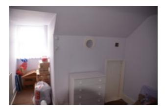
Where the separate WC is located at the uppermost level, the ceiling has been covered over in polystyrene tiles. These are regarded as a potential fire hazard and should ideally be removed. Upon removal it is likely that the ceiling beyond will be damaged.
