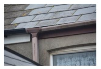
Guttering serving the side of the extension has been run in white half-round plastic sections. This too was seen to be in fair condition, there being a downpipe secured to the elevation wall by the store door, this ultimately jettisoning stormwater into the nearby gully, which also collects waste water from the bathroom. It was noted that the fixing bracket at the base of the downpipe has worked loose.
