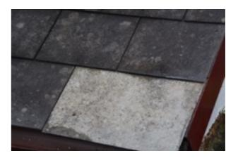
The roof slope facing towards the side yard was also seen to be in fair condition and free from damage or defect, but again a further small amount of moss growth was noted to be present.
