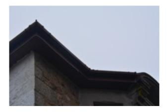
The final section of guttering is positioned to the right hand side of the bay where there is a further downpipe, this ultimately jettisoning stormwater into an open, although protected, gully at the base of the wall. It was noted that some of the cement benching surrounding the gully has now washed and weathered away, and this should be repaired to prevent water soaking down through into the foundation areas, which will ultimately cause damage and settlement problems.
