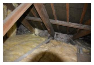
The very limited inspection of those parts of the void extending down the side revealed no obvious defects, with the roof again for the most part being clean, tidy and reasonably well insulated, to include for vertical insulation against the stud wall where the upper attic room has been formed. Where the chimney stack rises up on the gable end wall brickwork was visible, and this was seen to be in fair condition with no evidence of any rainwater penetration down through the uppermost parts.
